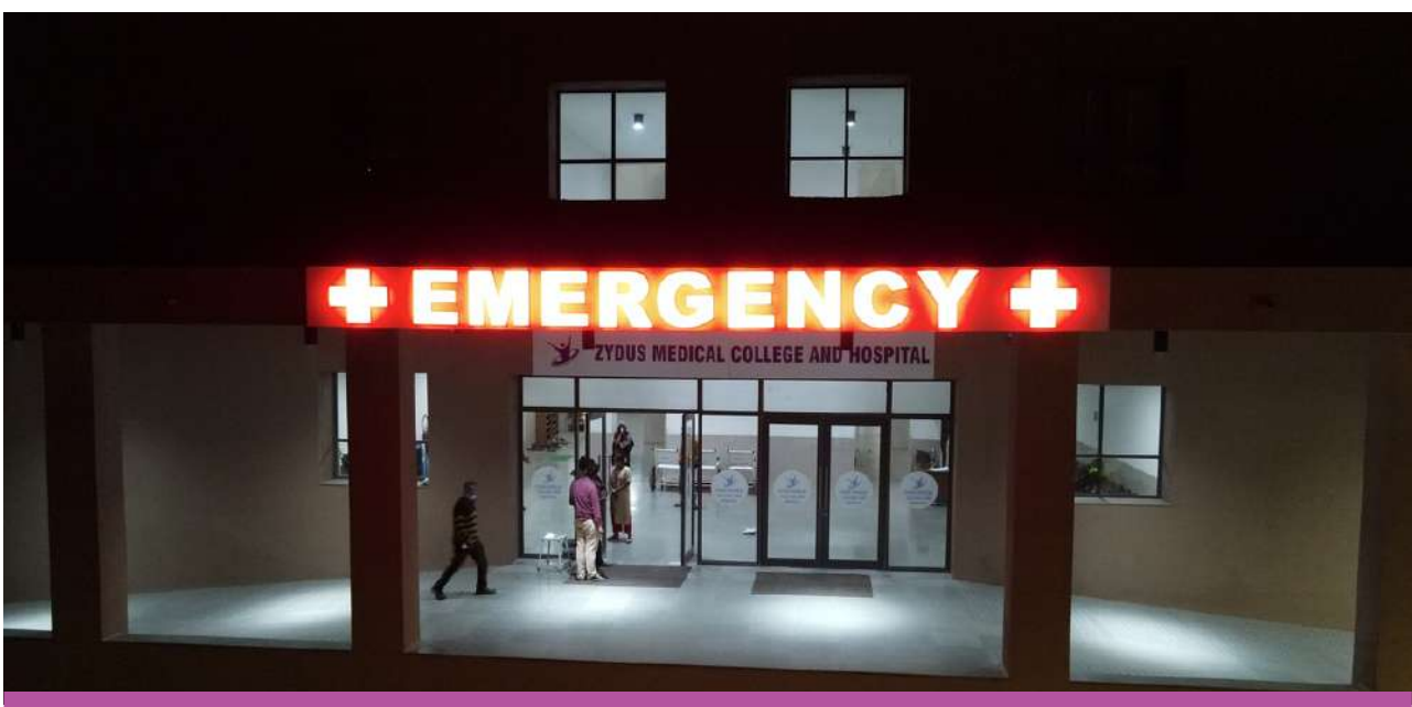
Emergency ward, ZMCH
