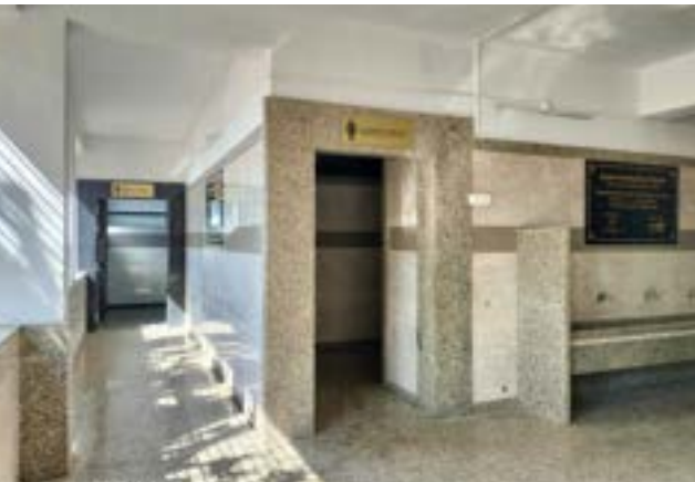
Toilet Blocks Constructed during Project Period
